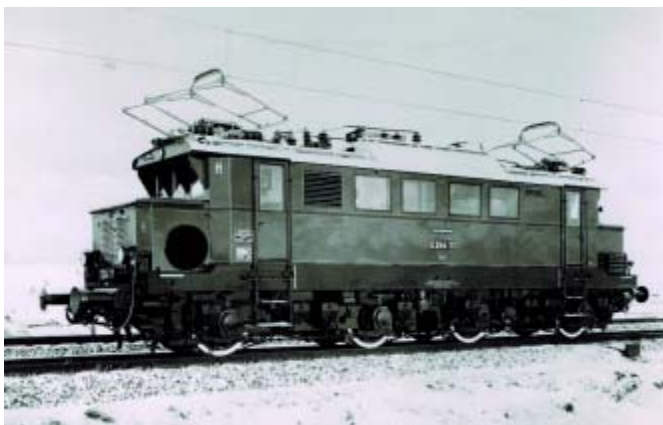
Figure 3 First locomotive using multi-anode mercury-arc rectifiers from BBC Mannheim, Germany (1938)
