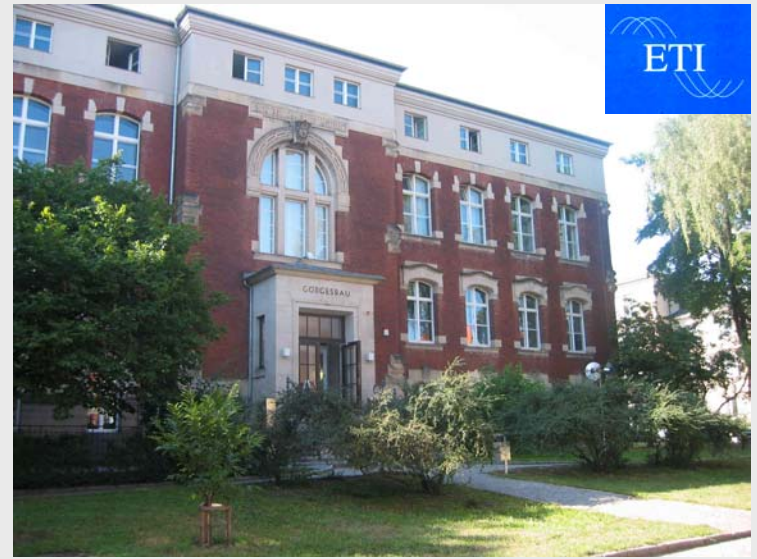
Görgesbau (Electrical Power Laboratory - ETI)
