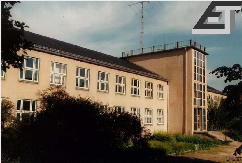
Barkhausenbau (Deans office and laboratories)
